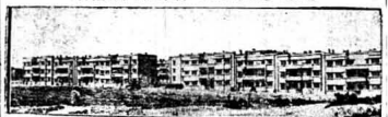
A row of new apartment houses for workers in the Soviet Union. In the Soviet Union, a workers country, the workers got the best and newest houses. There are no bosses owning the mills and factories in the Soviet Union.
